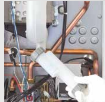
Removal of condensates siphon
