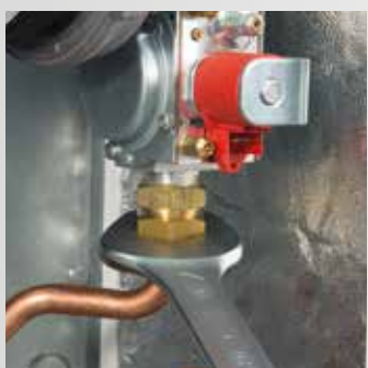
Removal of the fixing system on the gas valve
