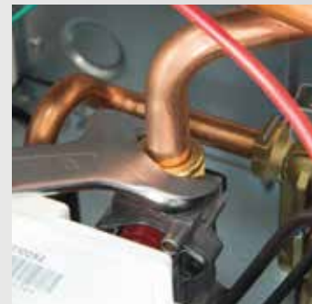
Removal of the fixing system to the pipeline
