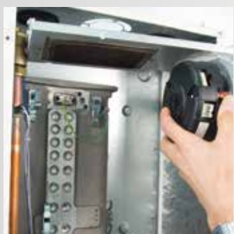
Removal of the complete combustion system
