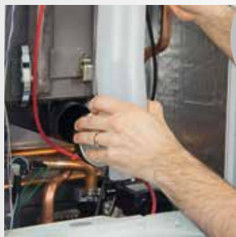
Removal of the smoke manifold
