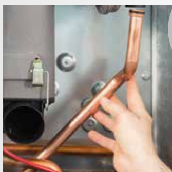
Removal of the gas pipe
